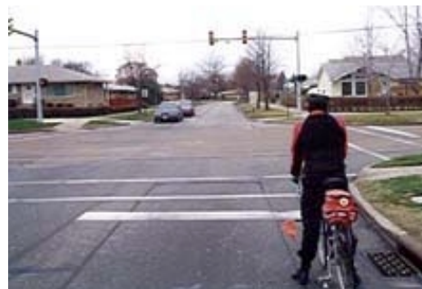
Simple Loop Detector: Detector wires are under the cyclist's left foot and also near left side of lane. (He should be further left.)
